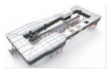
featuring a highly modifiable test section that can be adapted to a wide range of equipment and instruments. The Large Low-Speed Wind Tunnel, developed in 2019, houses an Aerodynamic Test Section and a Boundary-Layer Test Section, facilitating comprehensive General Aerospace Research and Civil Engineering Aerodynamic Testing including but not limited to structures like buildings and facades.
