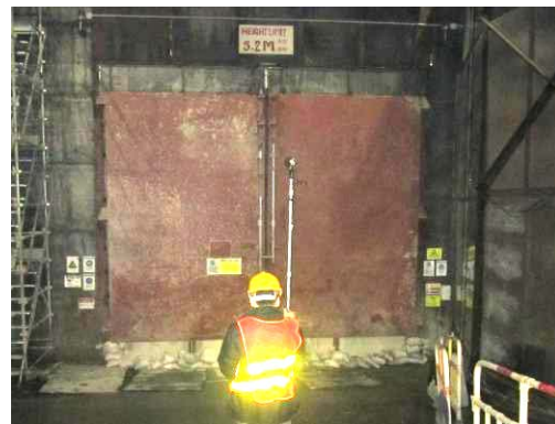
Photo 4: Tunnel acoustic at Pat Heung
